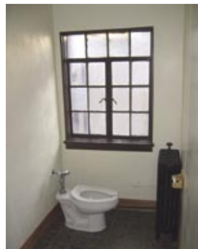
The Pope Suite bathroom was renovated earlier this year.
