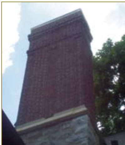
Picture of one of the redone chimneys
